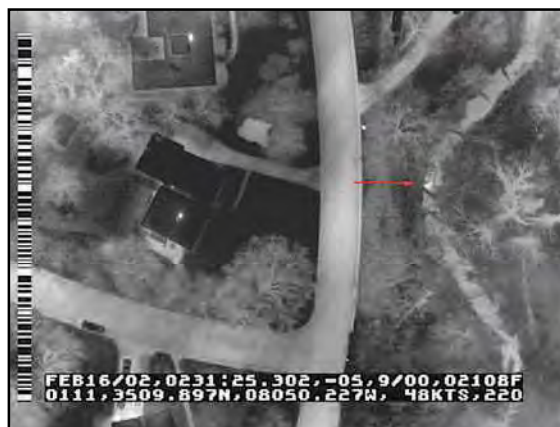
Figure 72: Aerial thermography showing sewage leak
