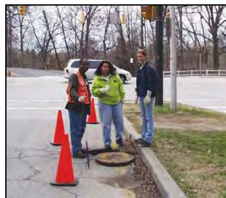
Figure 54: Traffic cones divert traffic from manhole inspection area
